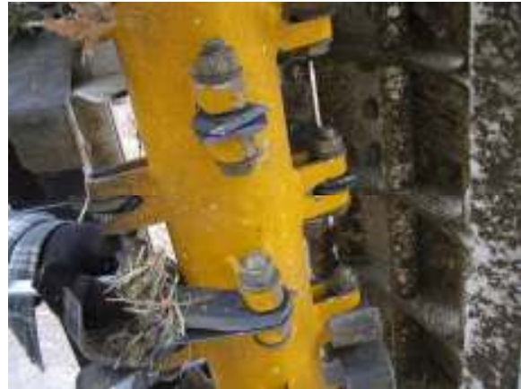
Figure 4: Broken Pre-Test Cutters
