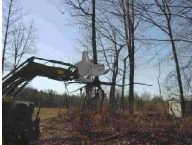
Figure 32: Tree Picker in Operation
