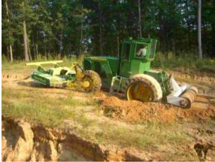
Figure 19: MCSV Stuck in Damp Sand Hill
