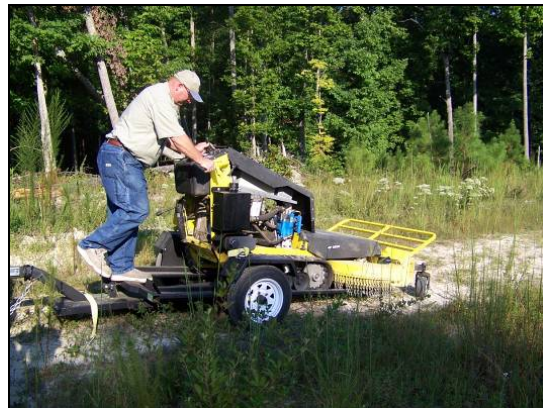
Figure 16: Loading Peco Cutter onto Trailer
