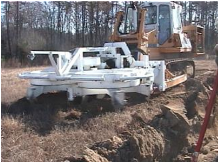
Figure 4. RMCT on Construction Dozer
