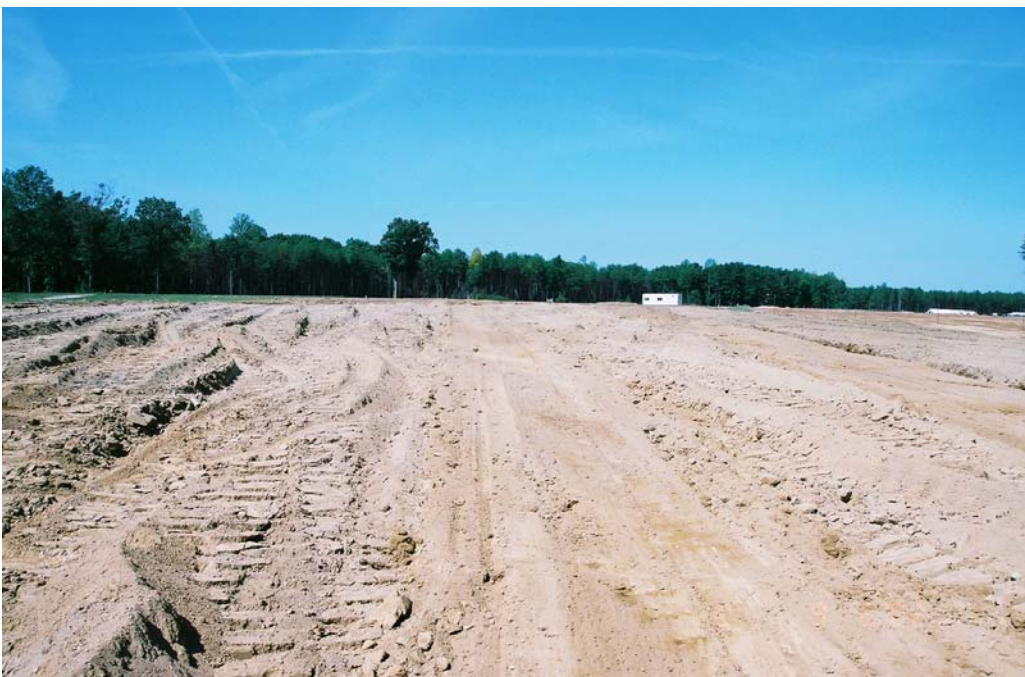
Figure 3. Tilled Area at Test Conclusion
