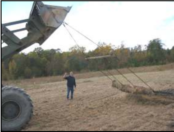
Figure 19. Clearing the MCR
